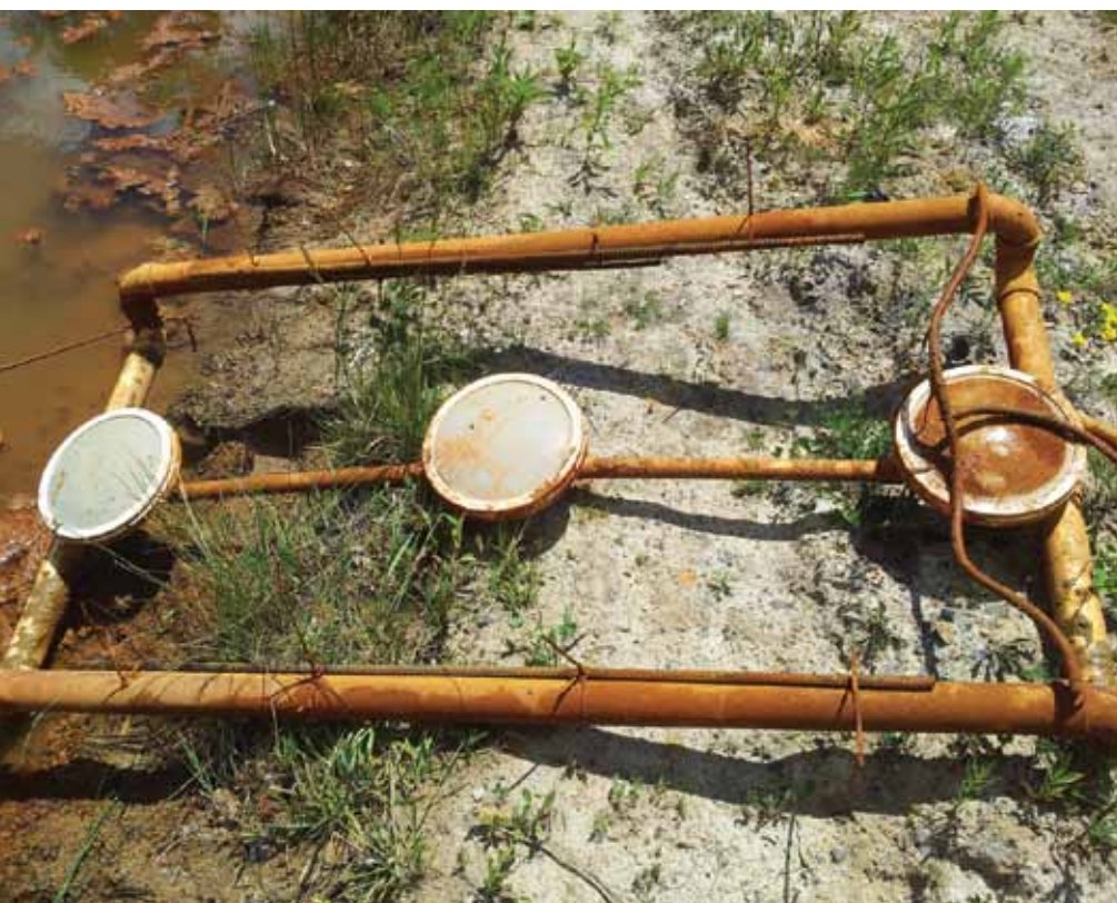
Figure 9. Fine bubble disc diffusers used at the Curley Passive Treatment System.
