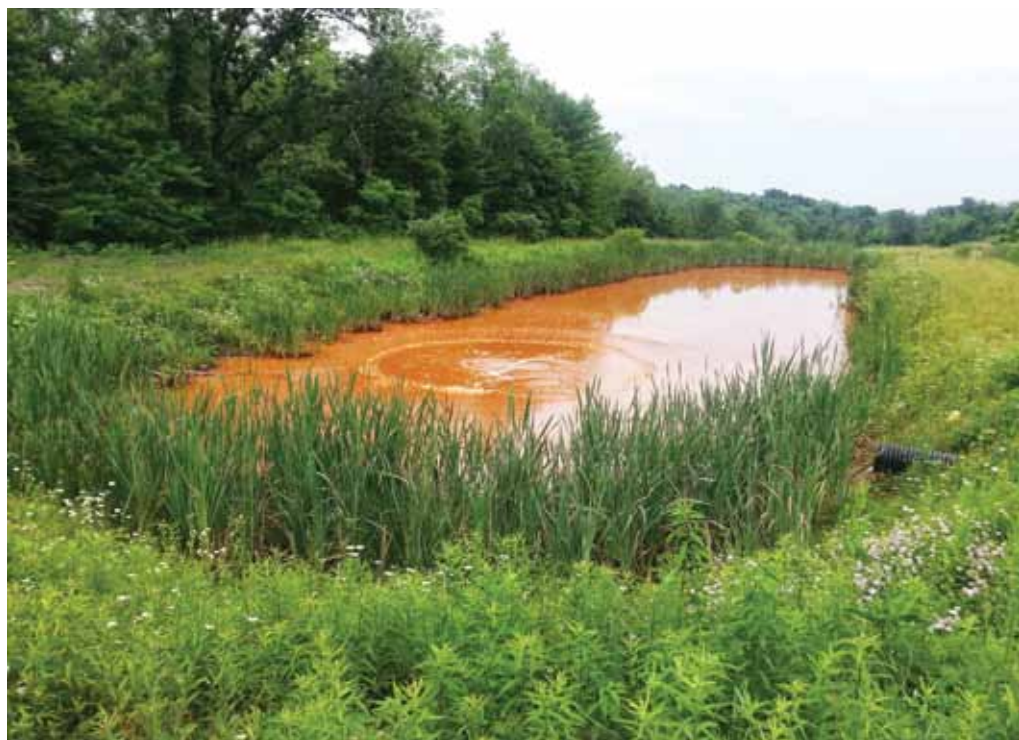
Figure 2. Aeration using a trompe at the North Fork Passive Treatment System.
